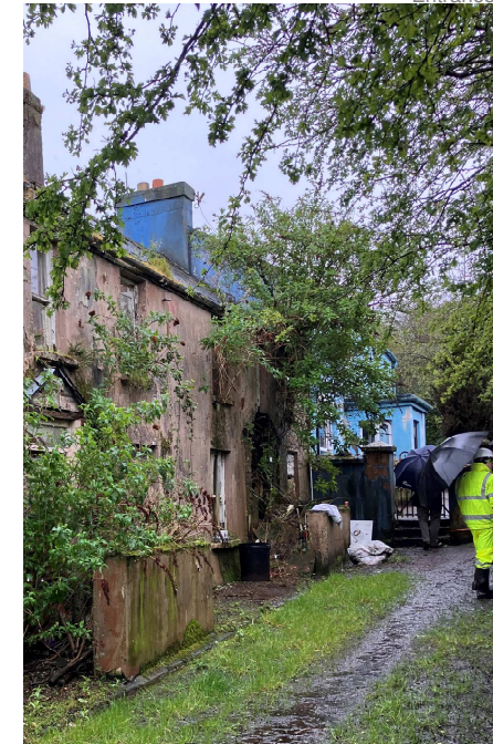
Condition of buildings on site
