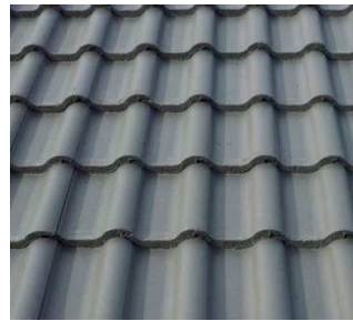
dark slate effect conc. tile to roofs
