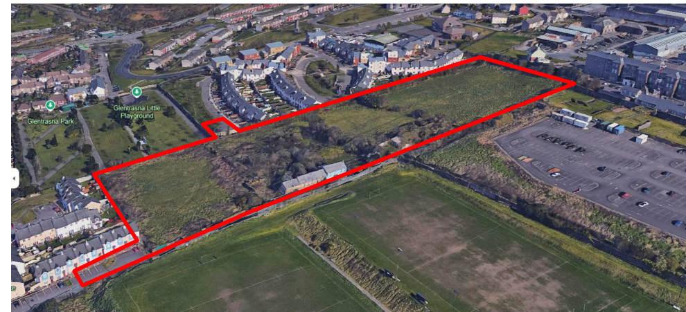
Aerial view of Pope's Hill Site.
