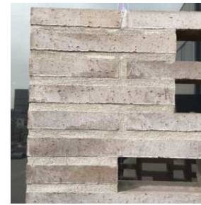
Flush pointed buff and red brickwork
